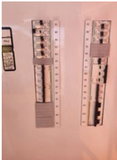
Image: Switchboard upgrades
