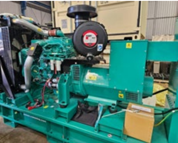
Image: Engine replacement
