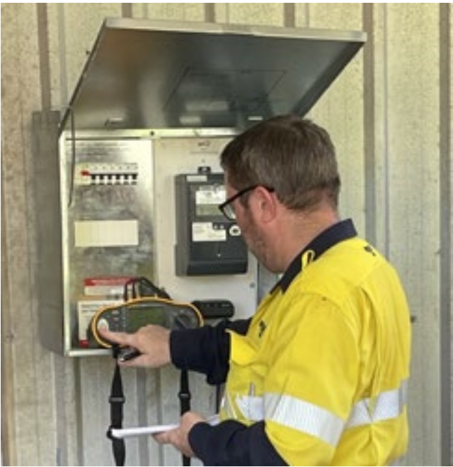
Image: AMI installation in Chile Creek
